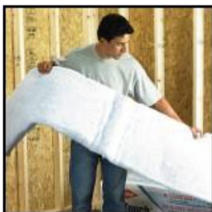
Dust and itch free insulation installation makes energy conservation more appealing.
