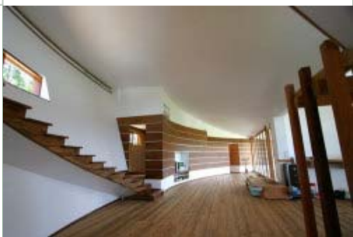
Shikkui natural lime plaster from Japan was used on the curving, unbroken interior walls of
