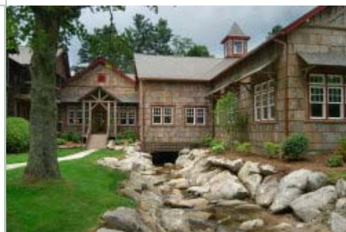
This addition to the Eseeola Lodge in Linville, North Carolina, completed in 2005, is sheathed with Bark House shingles made from tulip tree bark.
